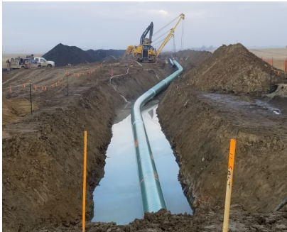
Description & Location: SF34 KP 966+476 Facing West Three side booms holding pipe for Denver Reid tie-in crew. De-watering crew pumping water from one end of the ditch to the other.
