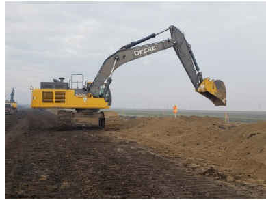
Description & Location: Photo facing North West SF 11 (KP 924) Excavator is backfilling trench.
