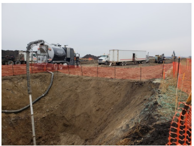
Description & Location: Photo facing South West SF 41A (KP979+400) Hydro vac removing water, Drill rig drilling under road.
