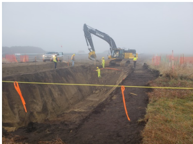
Description & Location: Photo facing West SF 10 West side of the road. Crew members using shovels to expose existing utilities.
