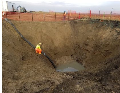
Description & Location: SF41A KP 979+410 Facing West Hydro-vac crew de-watering the ditch. Fences are in place.
